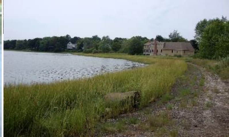
Mill Pond Way berm removal, 18 North Mill Pond, Portsmouth, NH
