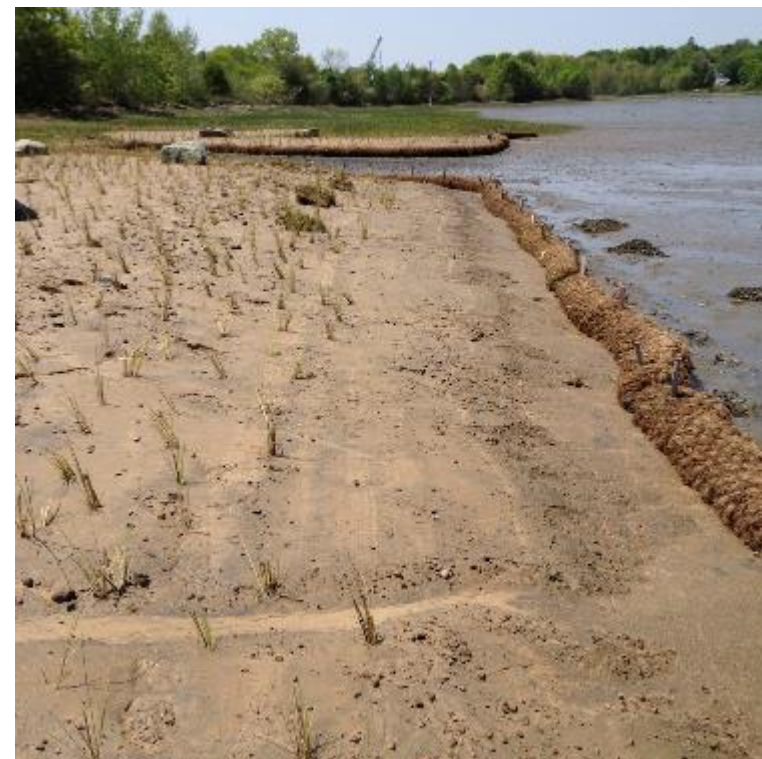
Brewster Street Mitigation on North Mill Pond (Stantec)
