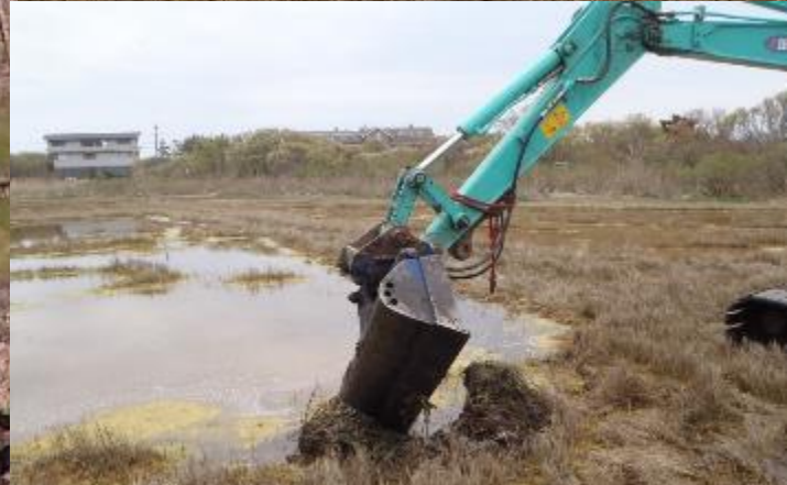
Runnels dug through ditch spoils
