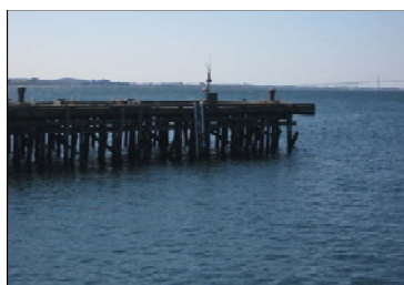
PVC deploying structure at T-Wharf
