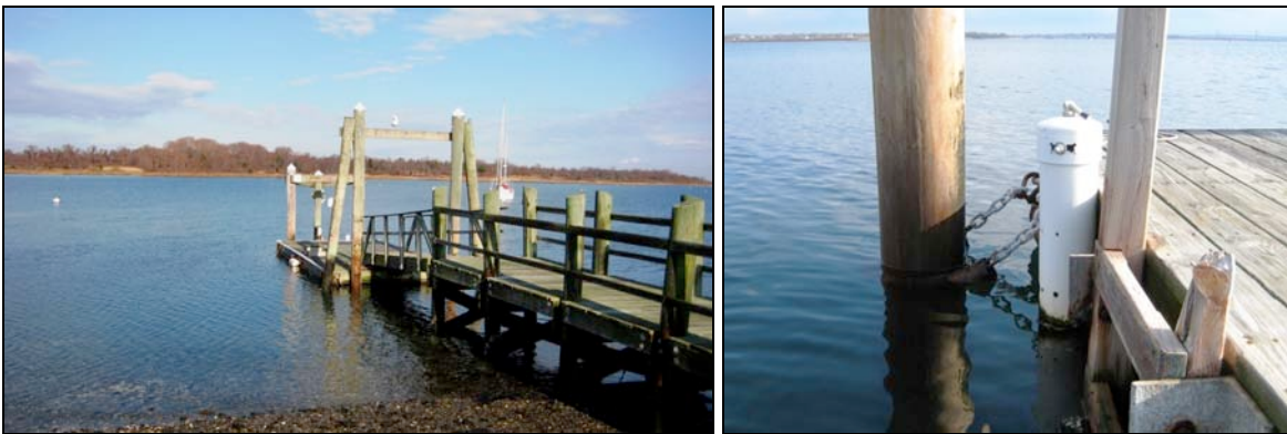
Figure 3. Potter Cove water quality monitoring station (left) and deployment structure (right).
