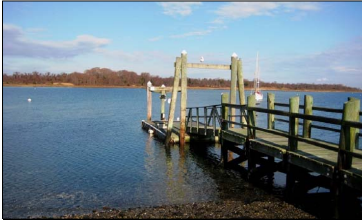
Figure 3. Potter Cove water quality monitoring station - the first SWMP station established on Prudence Island.
