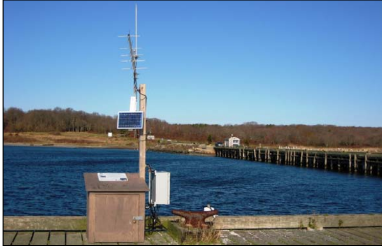
Figure 8. Telemetry station at T-Wharf transmits water quality data from the T-Wharf Bottom station via satellite. The near-real time data can be accessed online at http://cdmo.baruch.sc.edu/QueryPages/googlemap.cfm .
